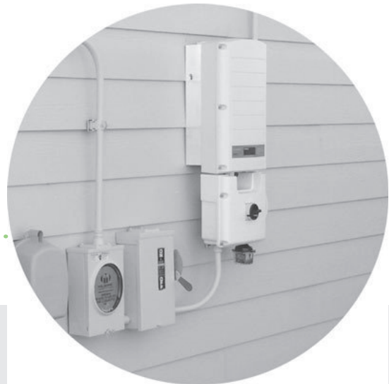
Figure 4: Close-up view of an inverter, meter and disconnect switch.
